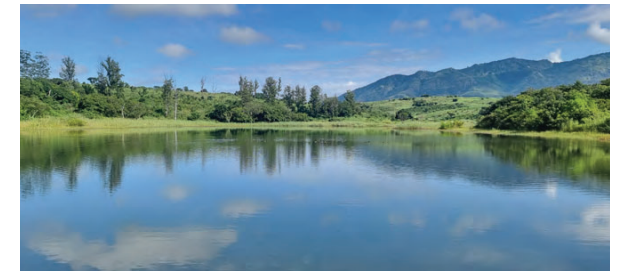
Cupi Dam, MML Mozambique: March 2024
